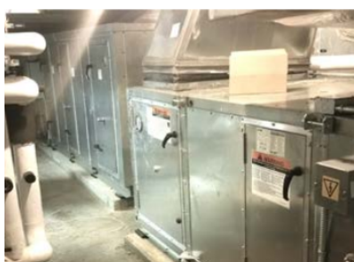
HVAC Renovation Bridge Point ES, Hill Country MS, Westlake HS
